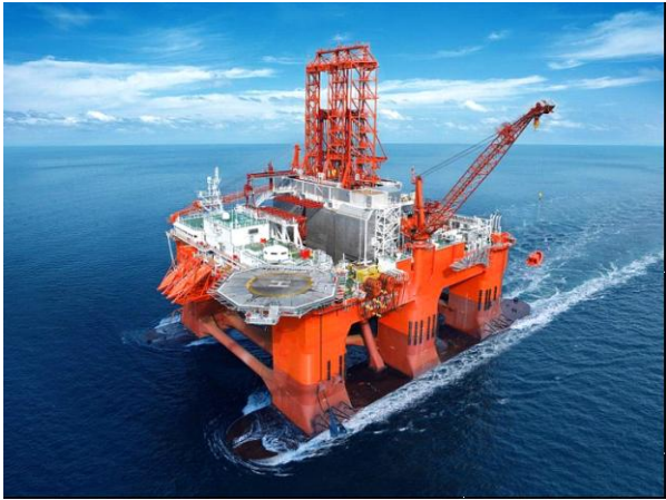
Figure 3: The West Phoenix drilling rig. (10)
