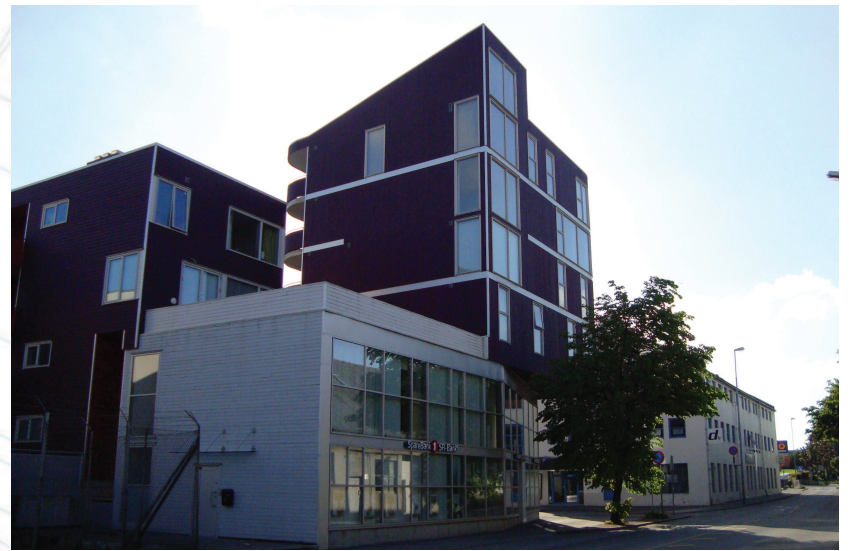
Img 5.8 The facade towards Haugesundsgaten
