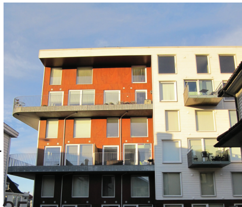
Img 5.5 Facade towards west
