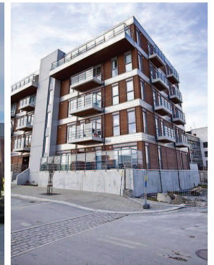
Img 5.13 Facade towards the water.
