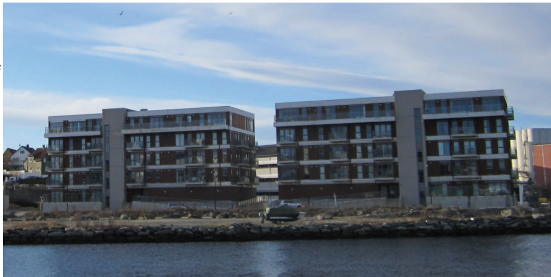
Img 5.12 The two buildings seen from Lervik Brygge project area.
