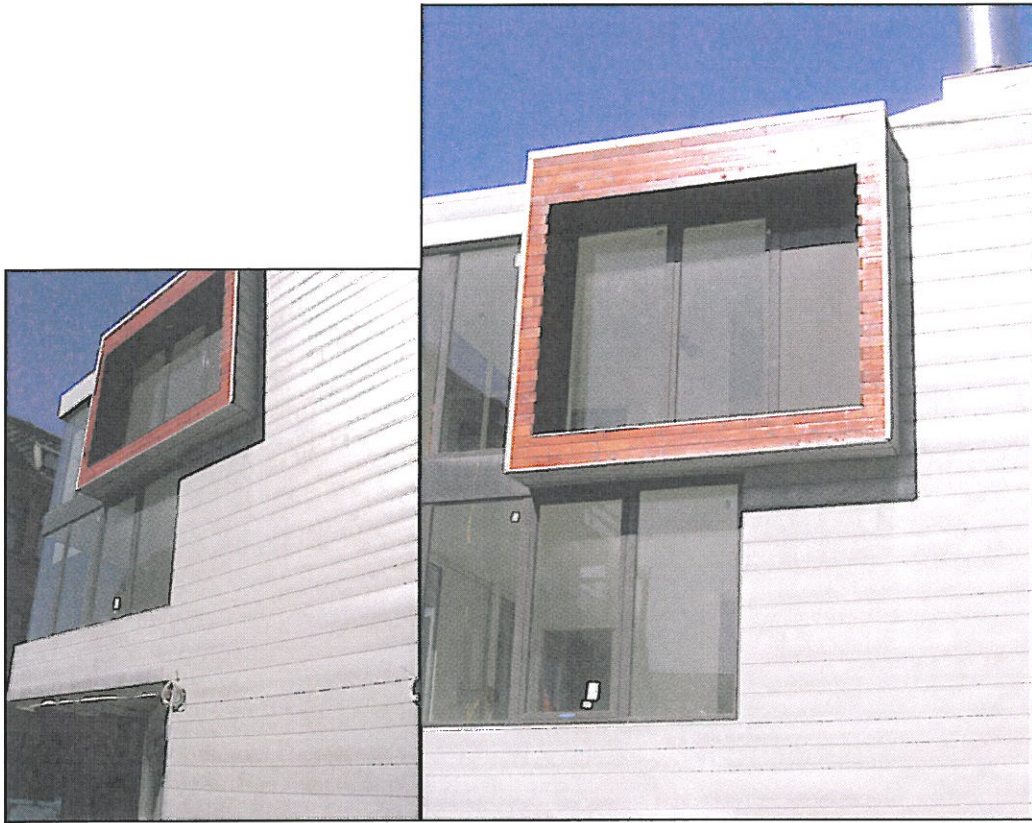
Photo 56 Reference to material usage on site
