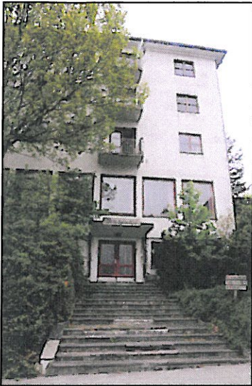
Photo 19 Previous canteen building at mental hospital
