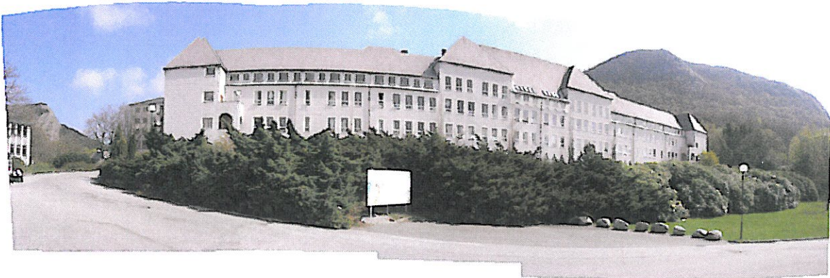
Photo 11 Main building, dormitory
