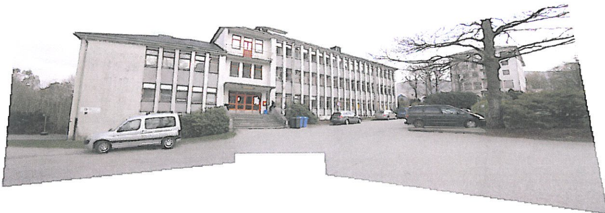
Photo 47 Close up north wall, car park to right
