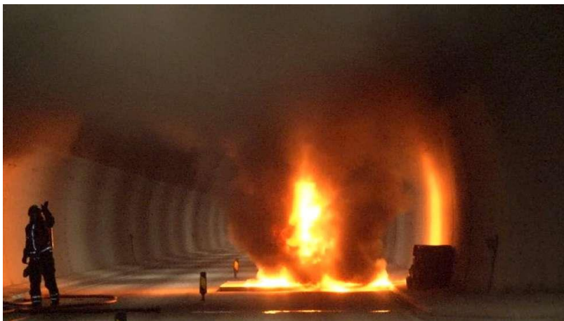
Figure 8: Fire in the Hell-tunnel (Photo: Frank Lervik, Adresseavisen)
