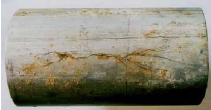
Figure 2.11. Stress corrosion cracking on 316L stainless steel (Energy Institute, 2008)
