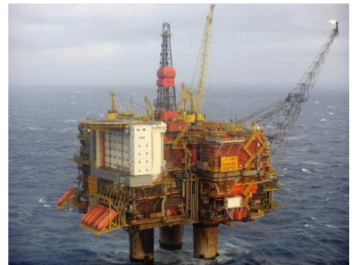
Picture 4: Statfjord A platform (20)
