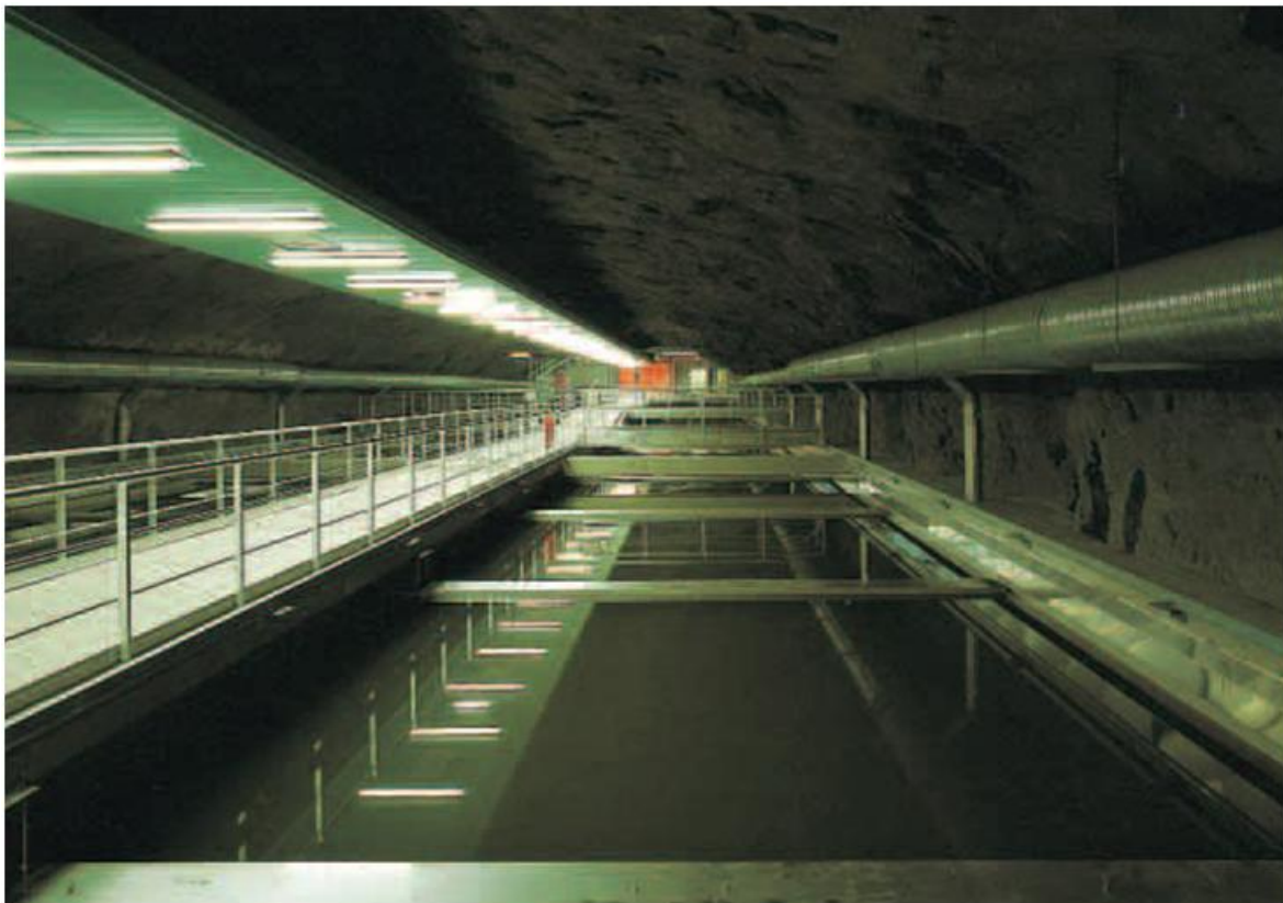
Figure 1.7 Sedimentation basin ( www.ivar.no )
