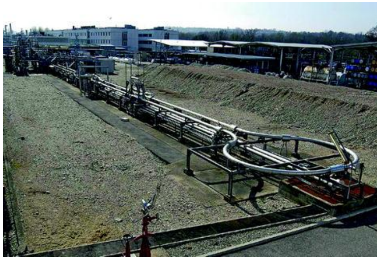
Figure 2.15 The “Lyre loop” multiphase flowloop for the study of hydrates in pipelines at IFP (French Petroleum Institute) near Lyon, France [19].
