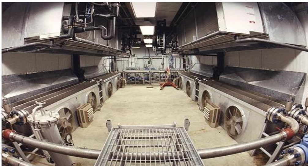
Figure 1.25. Flow loop 4inches (10,16cm) in diameter and 100m long.
