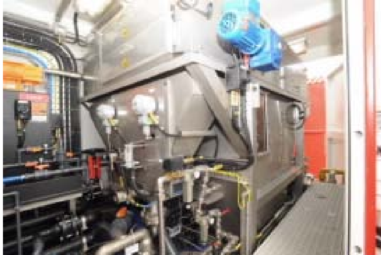
Figure 8: Sludge tank. [4]
