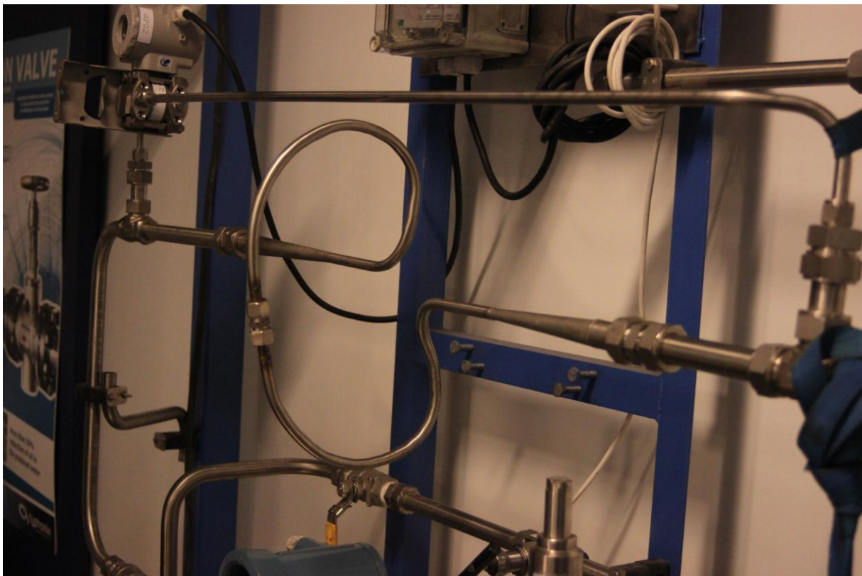
Figure 4-14: Cone (12mm) installed in the test-rig
