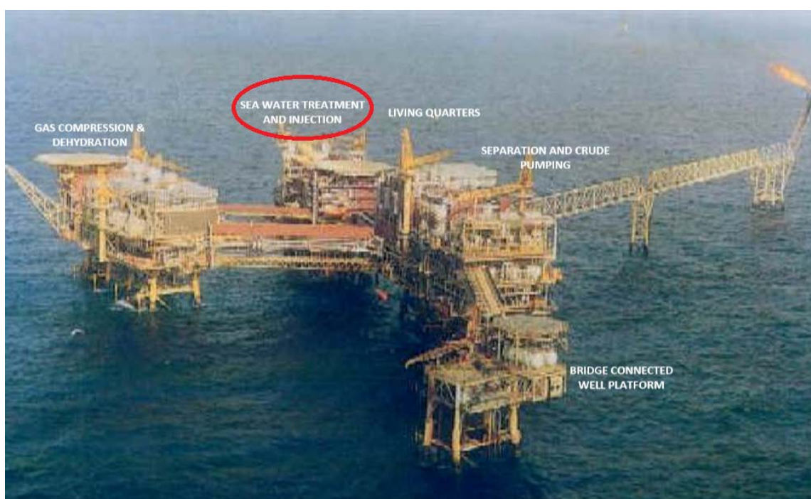
Figure 3.1: Water Injection Unit on Offshore Process Platform [Courtesy of ABB]
