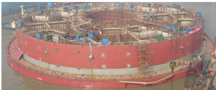
Figure 20.4: The SEVAN Driller under construction in COSCO yard.
