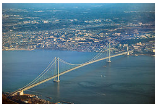
Figure 2.4.1: Picture of the Akashi-Kaikyo Bridge
