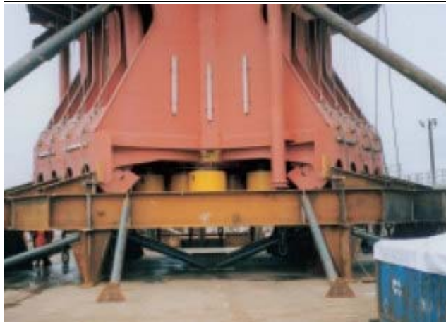
Figure 4: Plate girder grillage (Macswen, 2004)
