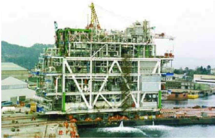
Figure 3: Skidding of a topside module to cargo barge. (Macswen, 2004)
