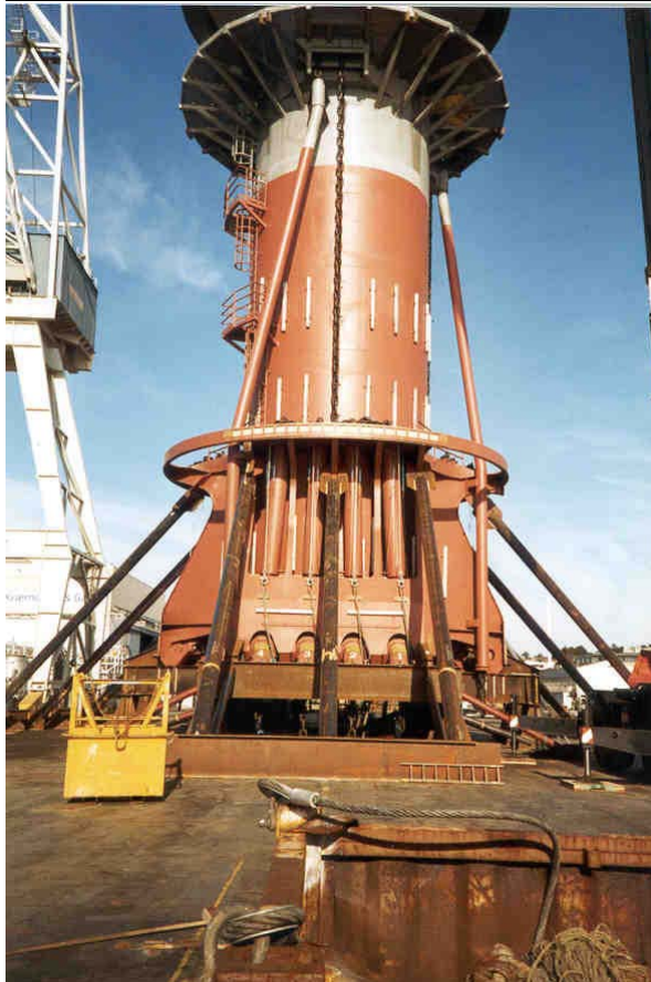
Figure 9: Example brace arrangement (Macswen, 2004)
