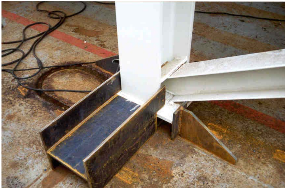
Figure 8: Simple shear plate securing. (Macswen, 2004)
