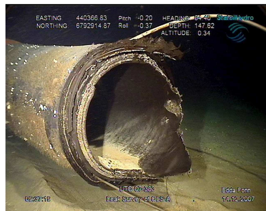
B) Picture of torn hose provided by ROV
