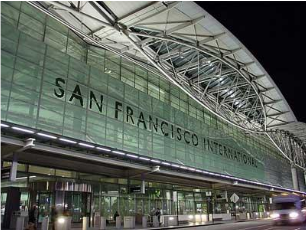
Fig. 2.14: The International Terminal at the San Francisco Airport. xxii
