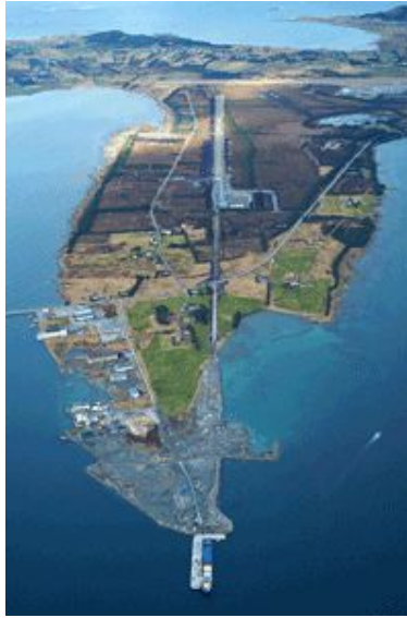
Figure 9-4 Pipes Onshore Fabrication – Vigra Spoolbase
