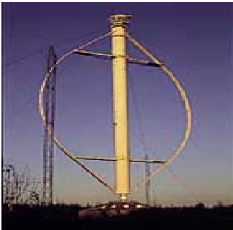
Figur 2.14 Darrieus Vindturbin [16]
