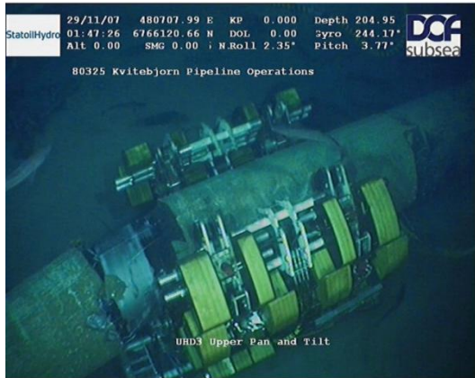
Figure 6-7. Coating Removal unit (CRU) to remove concrete coating. (Sources: Statoil)
