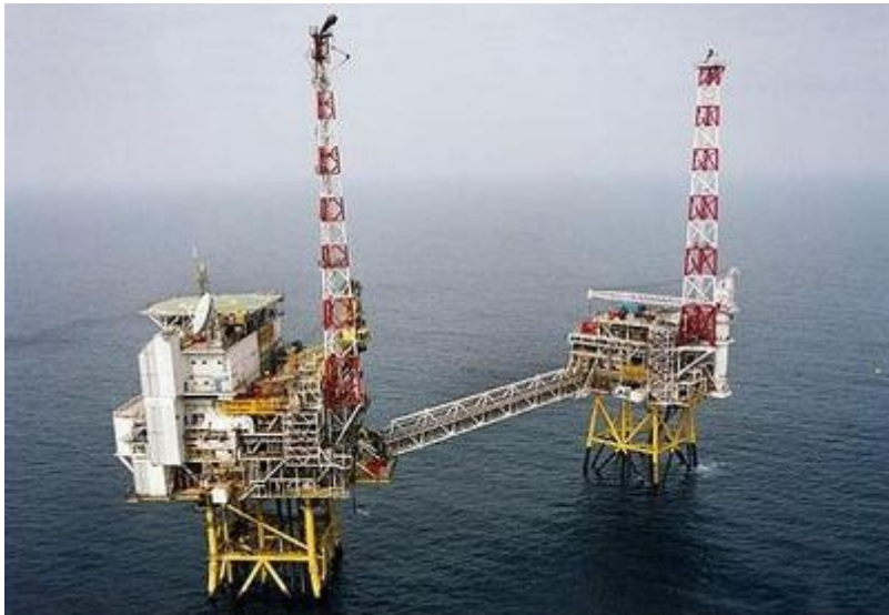
Figure 2.1 - Draupner E platform to the right.
