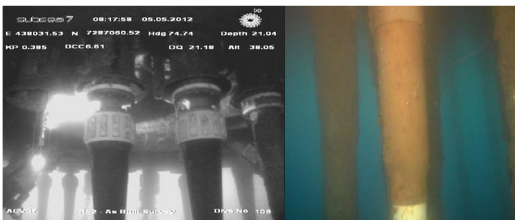
Figure 1-2: Left: The bend stiffeners protrude down from the I-tube at the hull of the Skarv FPSO. Right: A historical illustration of a loosened bend stiffener on an in-service FPSO (Subsea7, 2001 and 2011).
