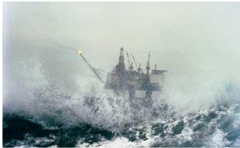
Figure 1 Offshore oil platform 'Gullfaks C' stands up to a fierce, North Sea storm [Husmo, A., 2012.]
