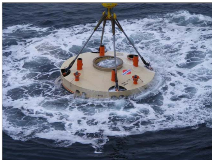
Figure 2-3 CAN being run through the splash zone [14]
