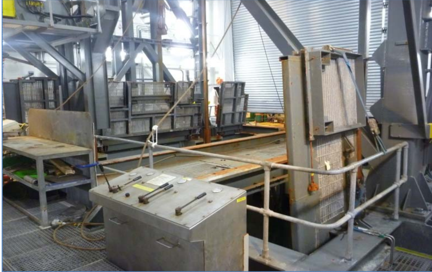
Figure 2.18 Moonpool hatch opening on Havila Subsea (Heng, 2012)
