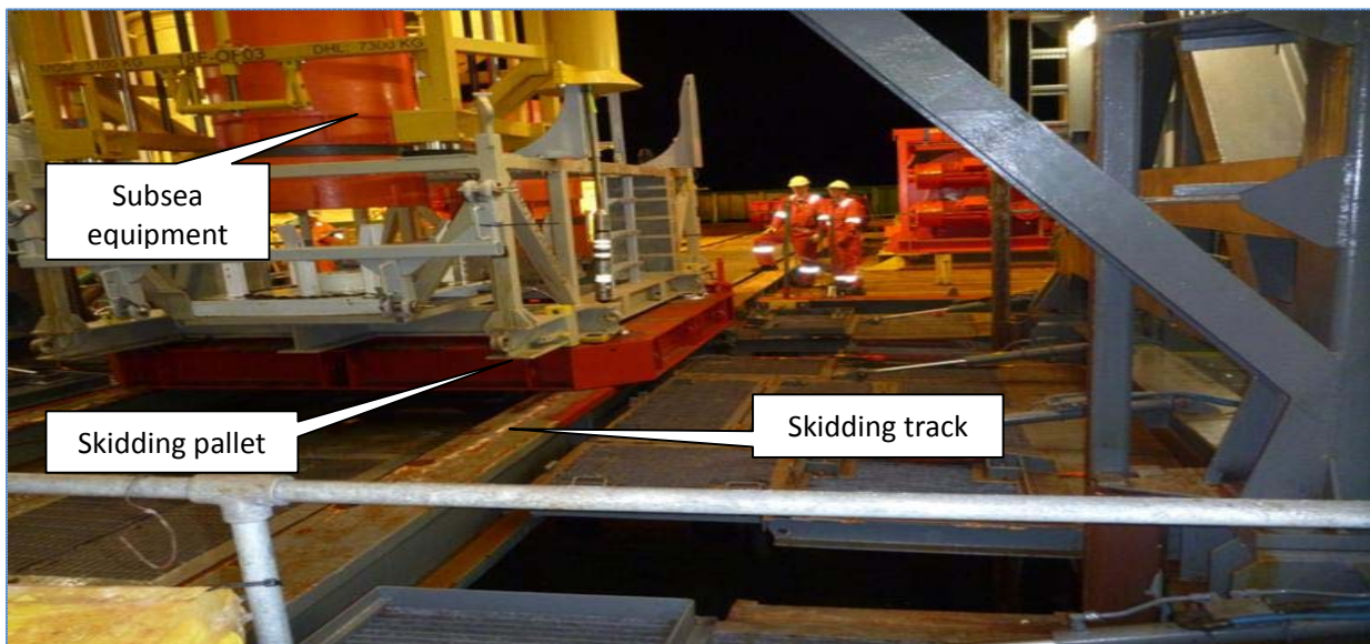
Figure 2.12 Skidding of Subsea equipment inside moonpool area on Havila Subsea (Heng, 2012)
