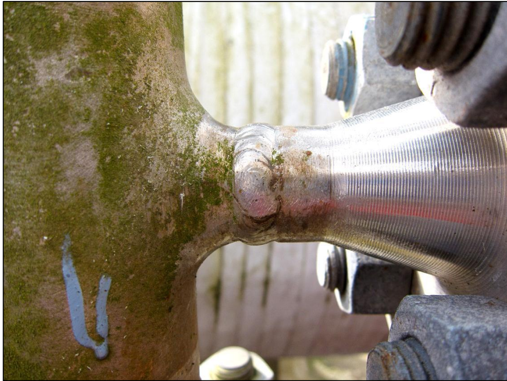
Figure 4-3 Detail of socket connected to CA-21-5111-FS20A in area A21
