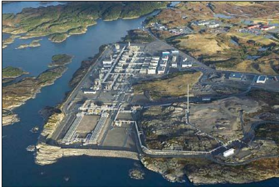
Figure 3-1 Kollsnes gas processing plant (Statoil 2007)
