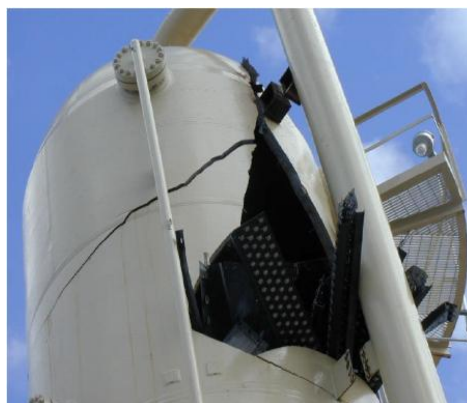
Figure 22: Ruptured pressure vessel shell.
