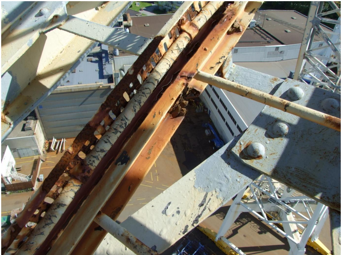
Figure 19 – an example of the corrosion on top of crane 520 Hensen (BGR, 2012)
