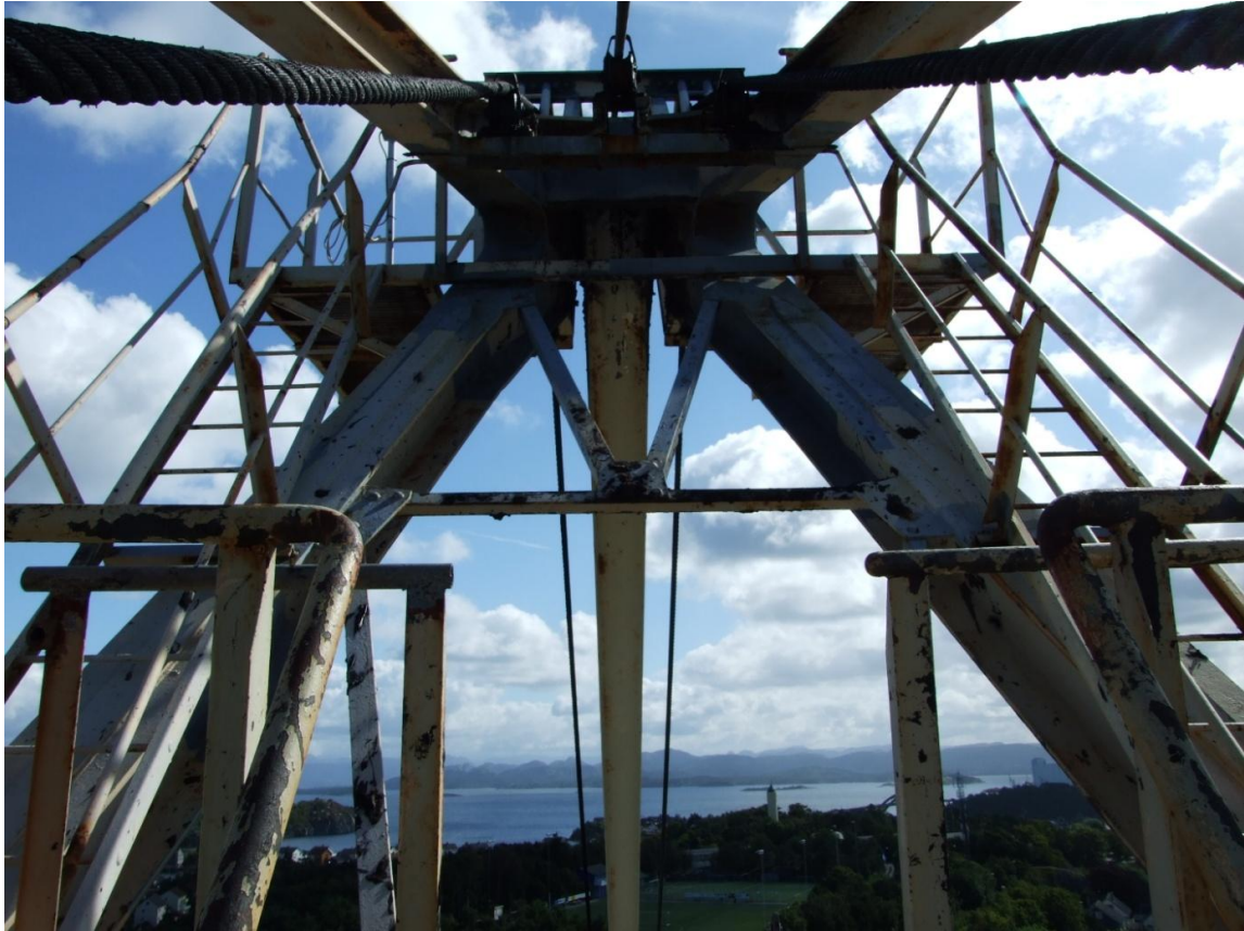
Figure 19 – an example of the corrosion on top of crane 520 Hensen (BGR, 2012)
