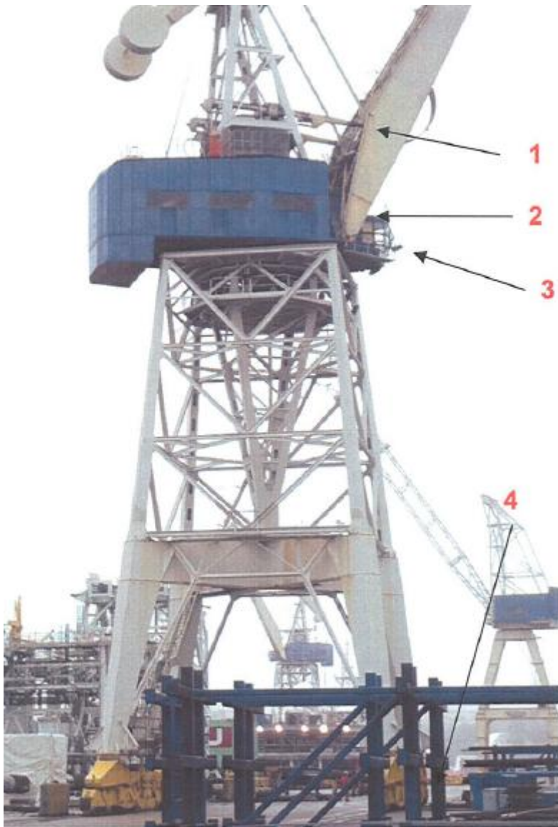
Figure 21 – Incident Crane 519 Hensen where a nut falls down from the tension rod (BGR, 2012)
