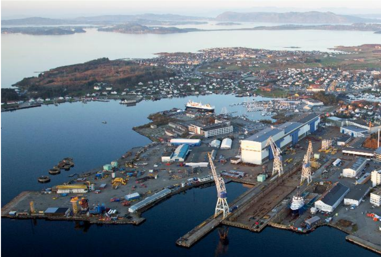
Figure 1 – Overview of Rosenberg Yard at Hundvåg, Stavanger. Here are also the three Portal Cranes shown. (BGR, 2012)
