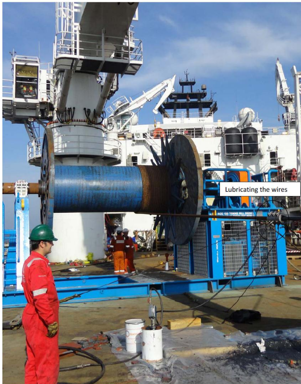
Figure 24: Lubricating the wires ( on construction vessel Skandi arctic)
