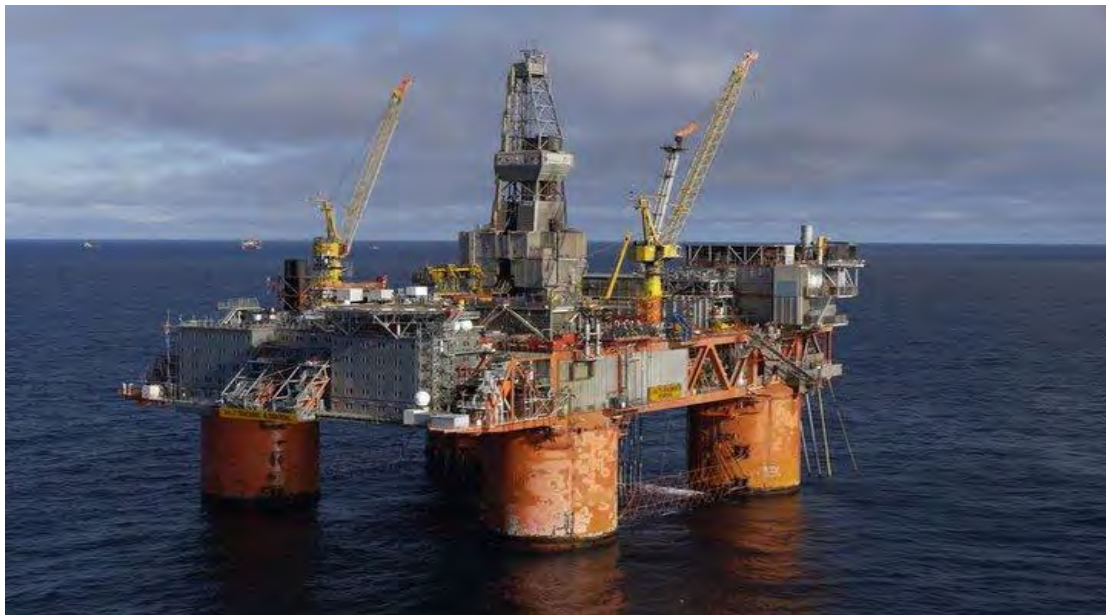
RIVING/INSTALL, Tie-in 24A/B.
