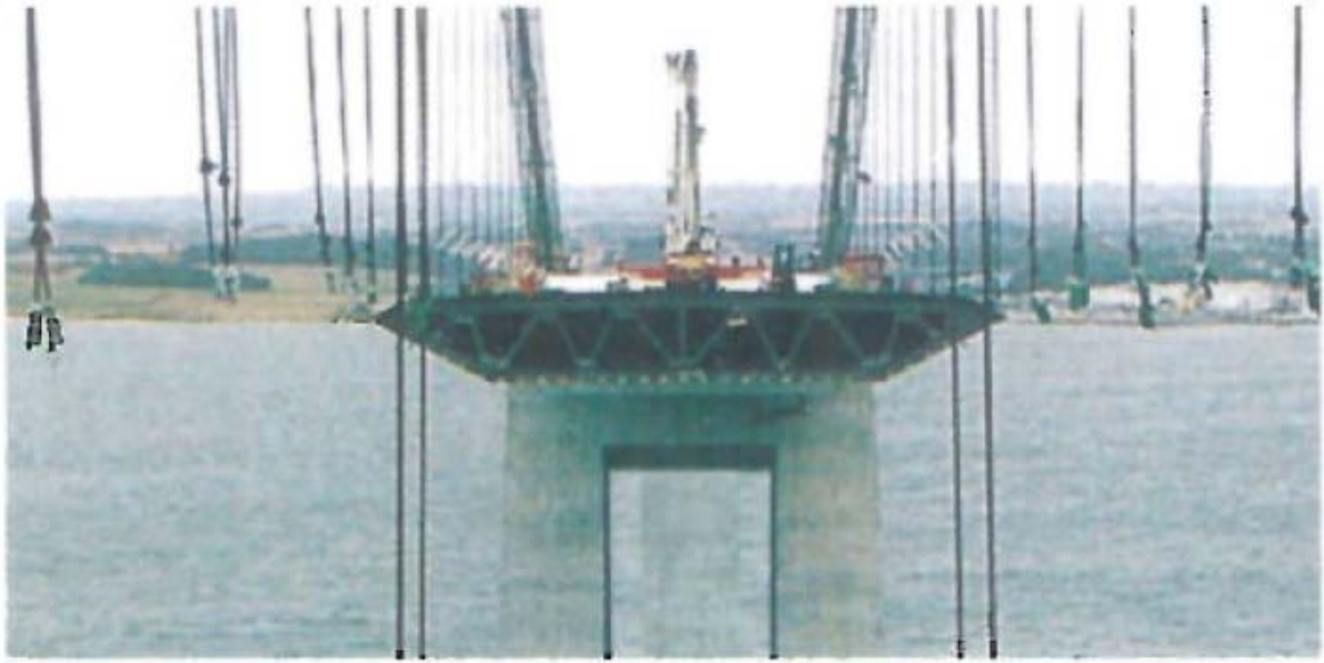
Figur 4-2 The streamlined bridge-deck of The Great Belt Bridge during construction [4]
