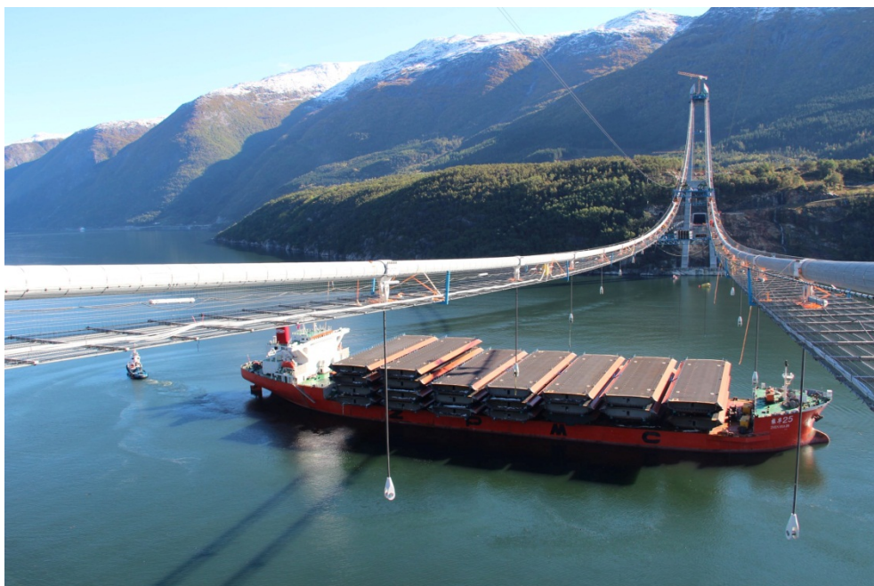
Figure 3-1 The Hardangerbridge - Stiffening girder prior to installation [13]
