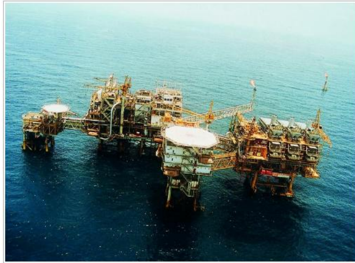
Figure 1.1: Topside Offshore Assets ( www.offshoreenergytoday.com )
