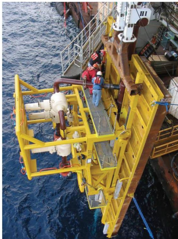
Figure 1.4 Inline Structure (Tee) Installation [6]
