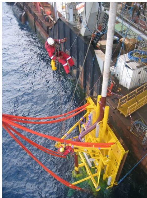
Figure 5.2 First End PLET Initiation [27, p.51]
