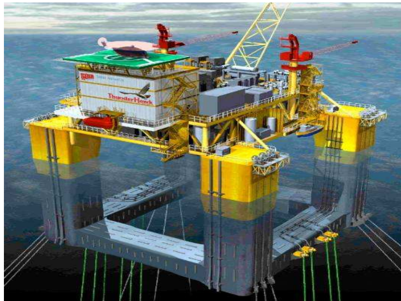
Figure 1-5 Polyester rope mooring Thunder Hawk Floating Production Unit ( http://www.offspringinternational.com/caseStudy/14/Polyester_Rope_Mooring_for_Thunder_Hawk_DeepDraft_Semi.html )
