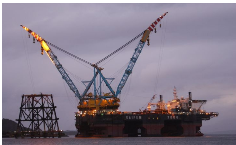
Picture 2-3 Saipem 7000 at Stord, Norway, [28]
