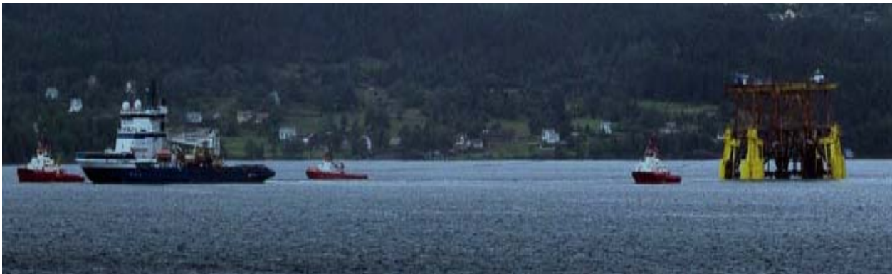
Picture 2-2 Tow of the DP2 jacket to Stord by use of the BTAs [24]
