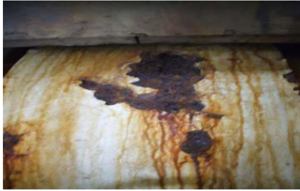
Figure 8: Coating Degradation
