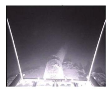
Figure 3-6 Kvitebjørn pipeline showing displacement caused by anchor (Gjertveit, et at., 2010)
