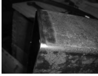
Figure 5.14 Spreader bar after treatment
