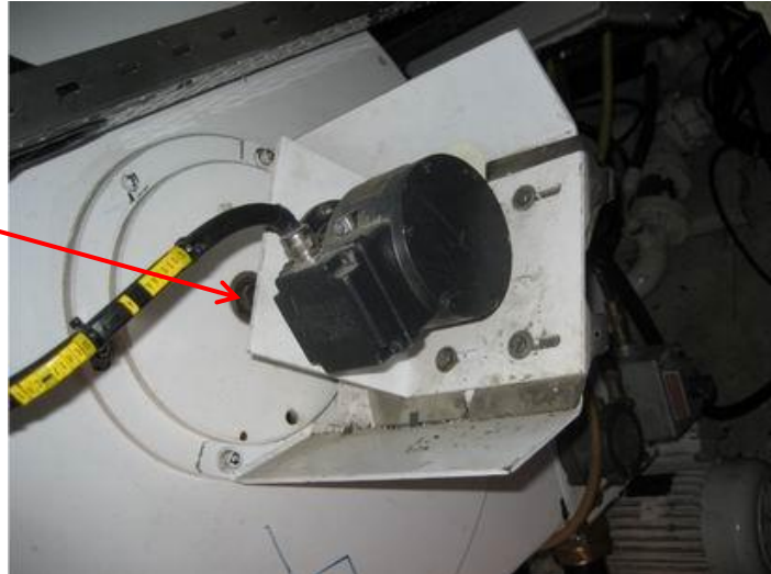
Figure 3.3 the coupling installation of Drawwork Encoder
