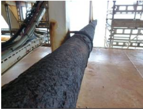
Figure 22: Picture of general rust build-up ca.10mm along the line
