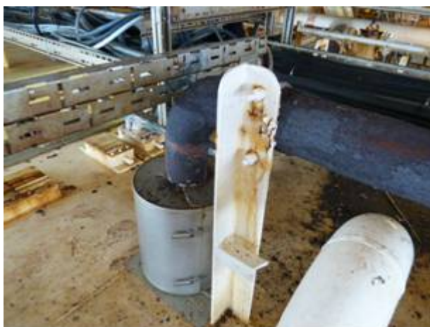
Figure 20: Reviewing the roof of the emergency generator room
