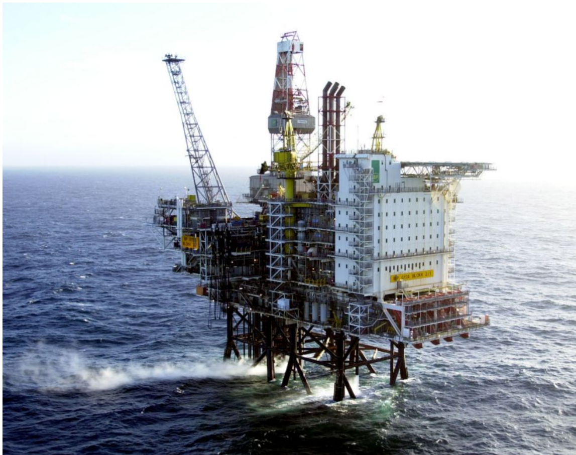
Figure 2.2, The Gyda platform.
