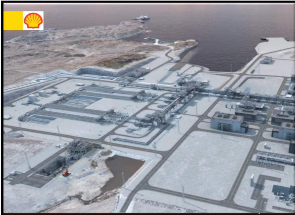
View of the onshore gas processing plant at Nyhamna – the subsea compression test site can be seen in the left lowermost corner. (Shell, 2010)
