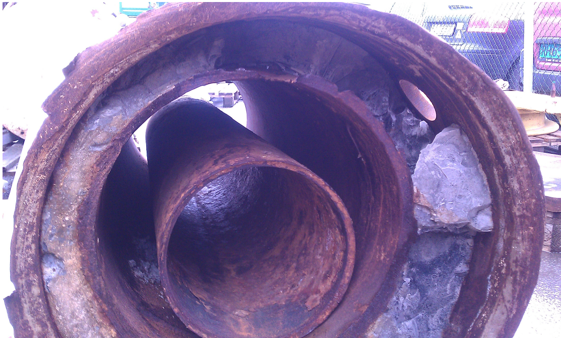
Figure 8: Multiple casing cut
