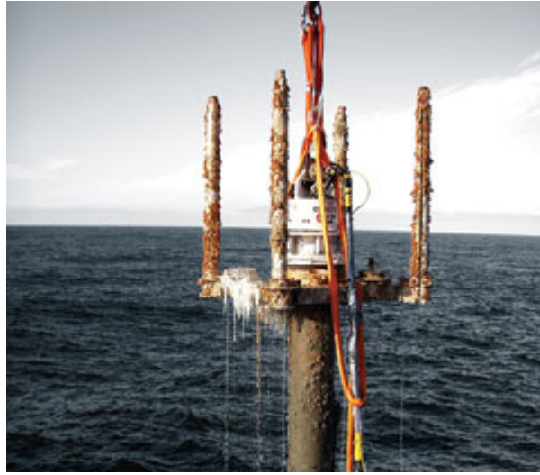
Figure 46: Wellhead and multi string conductor removal. http://www.epmag.com/Production-Drilling/Decommissioning-Abandonment-Coordination-ensures-decommissioning-success_44547
