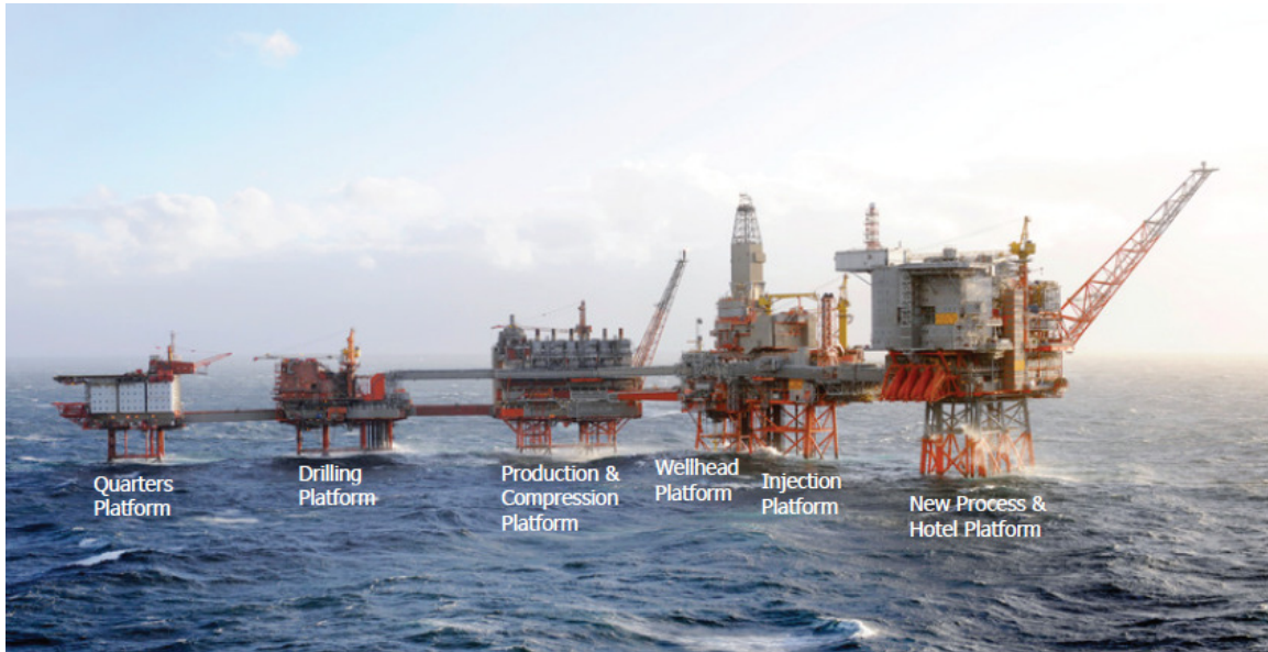
Figure 10: The Valhall field center. [2]
