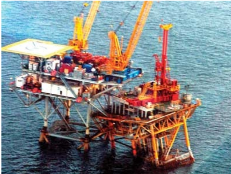
Figure 49: Pulling and Jacking unit placed on deck of damaged platform. [41]
