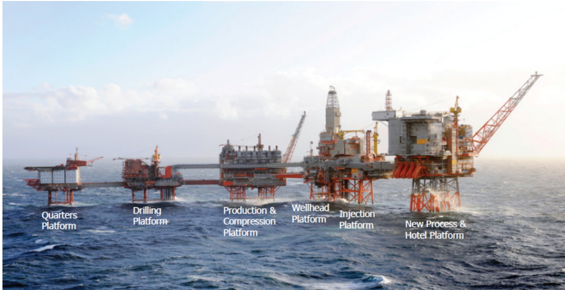
Figure 4: The Valhall field center. [2]
