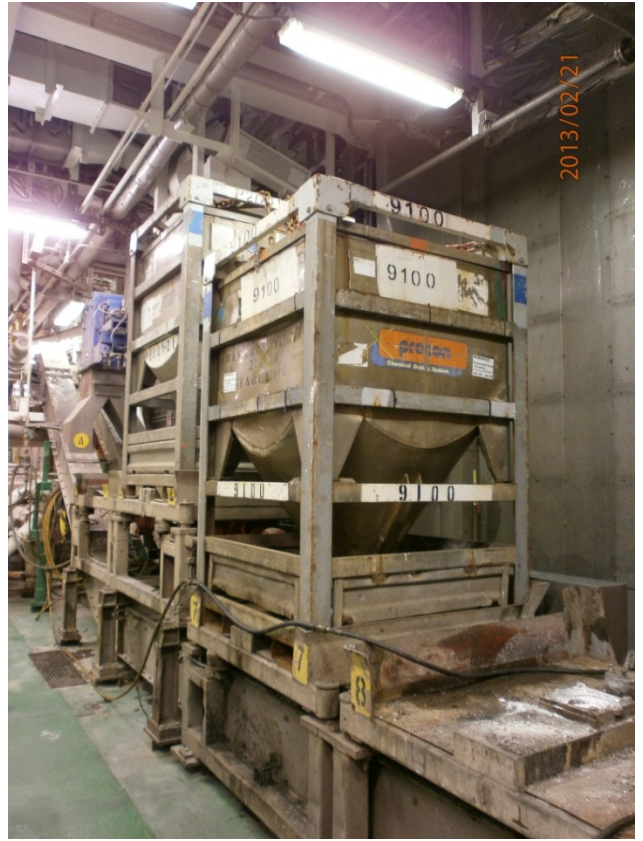
Two Procon tanks side by side
