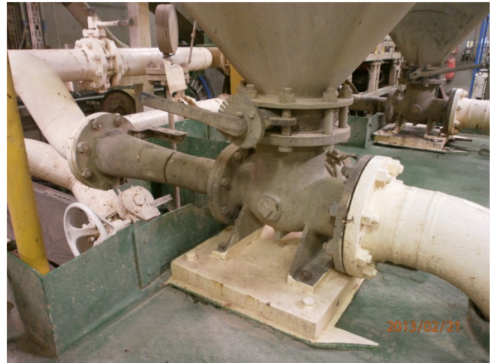
Detail of the venturi pipe of the hopper
