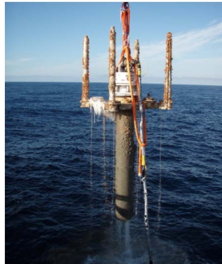
Figure 12 Wellhead removed from a well [29]
