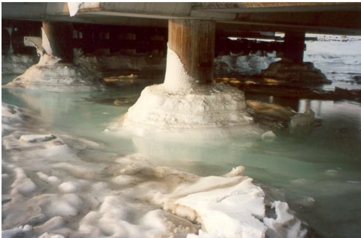
Figure 13 Freezing ice stuck to a pillar. (Løset and Marchenko 2009)
