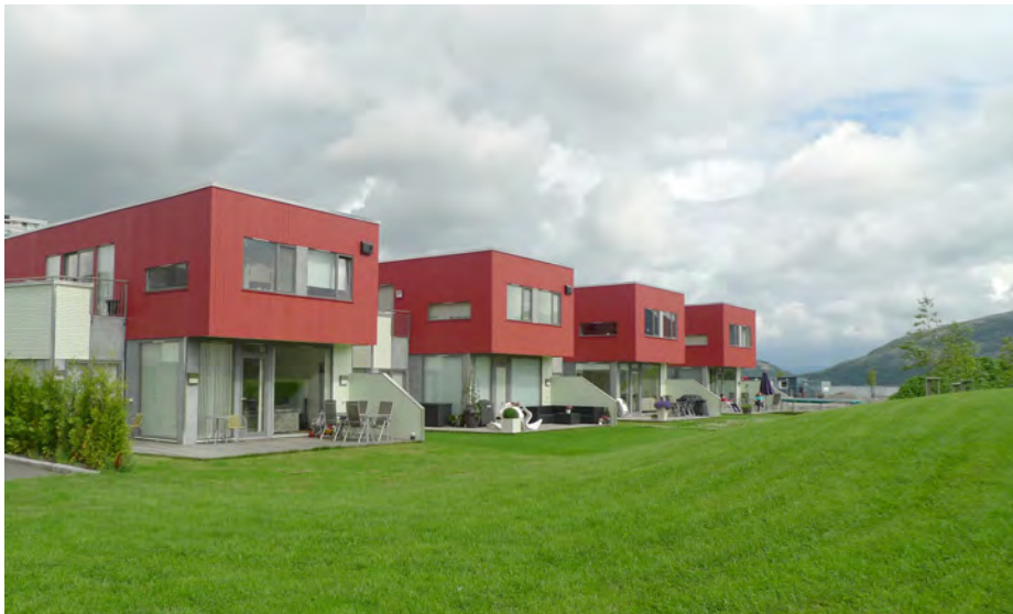
Four single family detached houses face the undulating lawn and open landscapes on the southern boundary of Jåttåvågen near Boganes.
