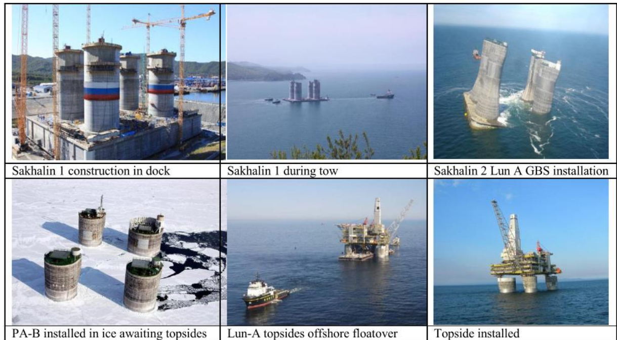
Figure 29 - Construction and installation of OIRFPs for Sakhalin projects 46
