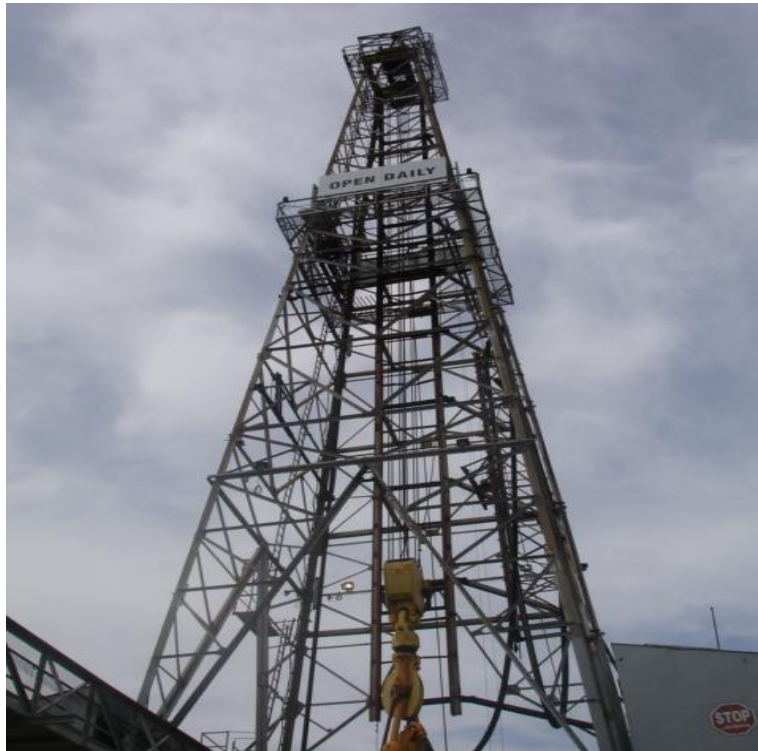
Figure 4 The derrick with a yellow traveling block
